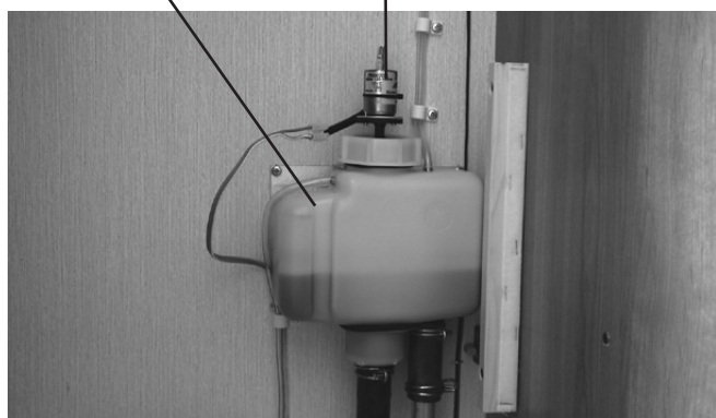
Expansionskärlet Cirkulationspump
