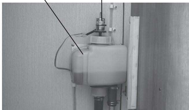
Expansionskärlet Cirkulationspump
